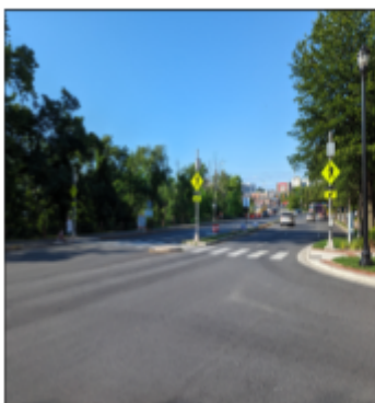
Example Rapid Flashing Beacon
